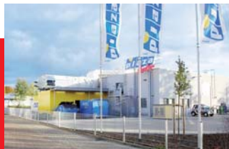
Left Entrance area
